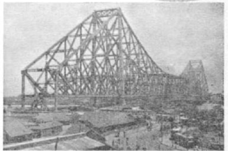
5. Howra Bridge - Calcutta.
